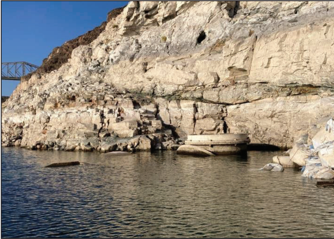
SNWA's Original Intake
