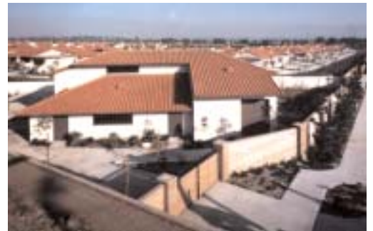
The Upland Hills Water Reclamation Plant in Upland, Calif., is an enclosed treatment facility immediately adjacent to a residential development. The plant has been in operation for almost 20 years.
