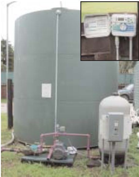
The storage tank and equipment for the demonstration project. (Inset) A separate irrigation controller.
